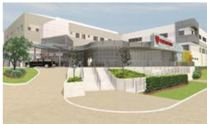
The new year marks the point of visible construction on campus.
